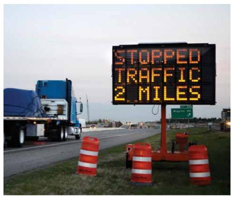
Overview Figure: Smart Work Zone/ITS systems have shown that they can reduce or completely eliminate rear-end collisions by reducing queuing, congestion and confusion by giving motorists information far upstream, away from the actual work. On this Texas roadway, a large truck reduces speed after the driver receives a warning of stopped traffic ahead. (Source: TxDOT)
